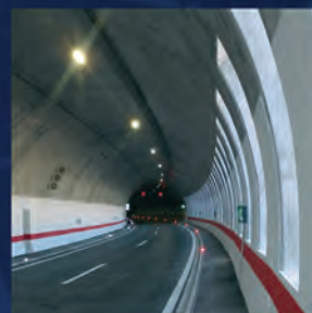
Tunel Sarani, autoput E 763: Beograd - Južni Jadran, Srbija Tunnel Sarani, highway E 763: Belgrade - South Adriatic, Serbia
