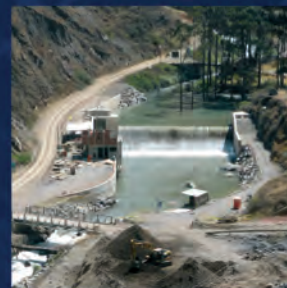
HE Chancay&Ruckuy, Peru HPP Chancay and Ruckuy, Peru
